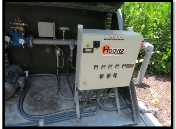
Figure 30 Irrigation Pump Station
